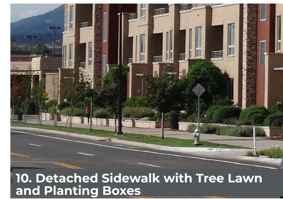
10. Detached Sidewalk with Tree Lawn and Planting Boxes
